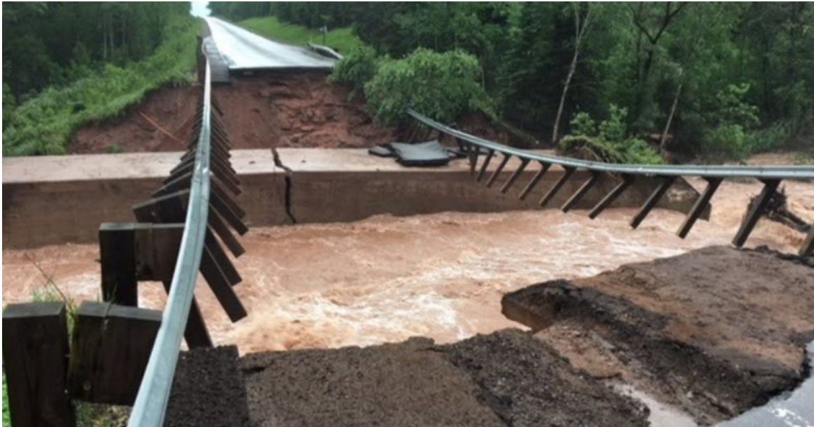
Figure 3.3.2-3: US Highway 2 in Bayfield County at North Fish Creek
