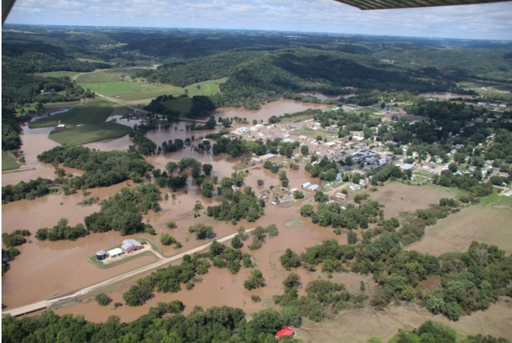
Figure 3.3.2-5: Flooding at La Farge, WI
