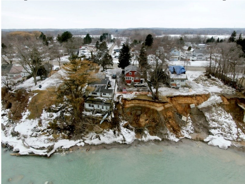
Figure 3.6.2-2: Lakefront Erosion in Somers Village
