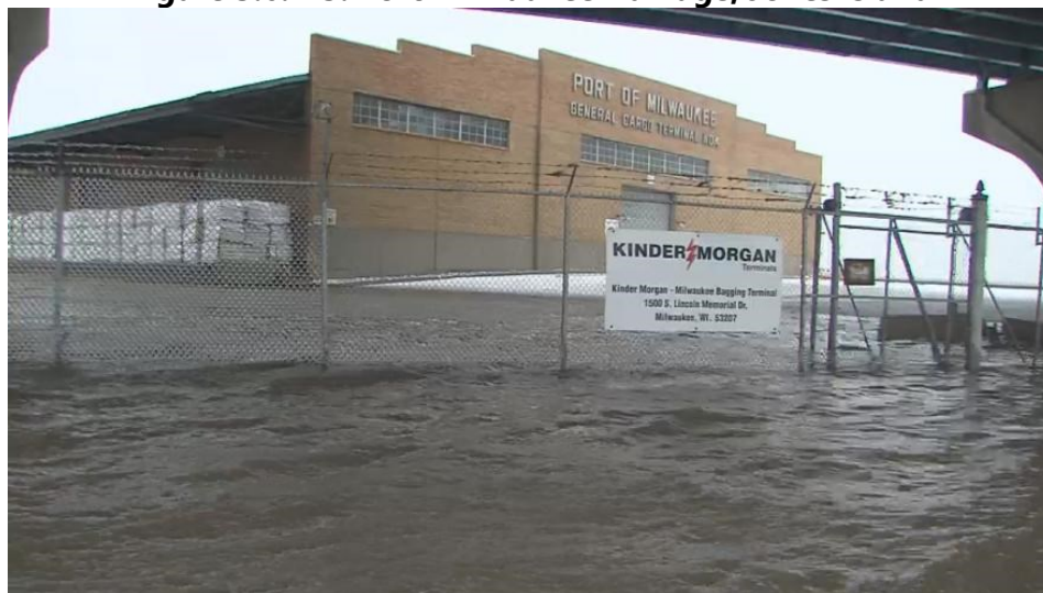
Figure 3.6.2-3: Port Milwaukee Damage, Jones Island
