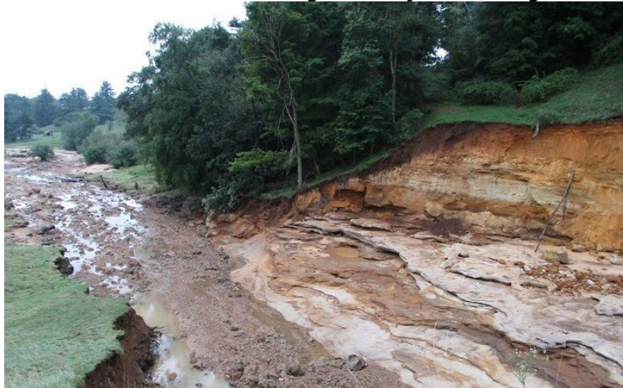
Figure 3.4.2-1: Mlsna dam following the heavy rains of Aug 27-28, 2018
