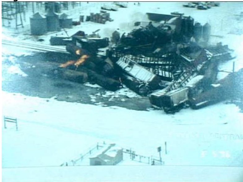
Figure 3.11.2-3: Overhead View of the Train Derailment
