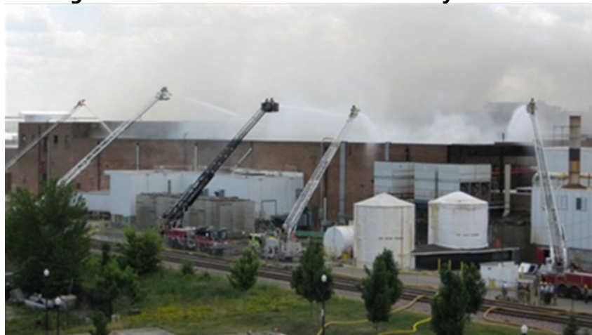
Figure 3.11.2-2: East Side View of Cudahy Plant Fire
