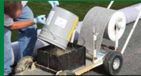
Gluing seams using seaming tape and glue box
