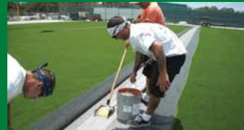
Gluing seams using stand-up trowel and seaming tape
