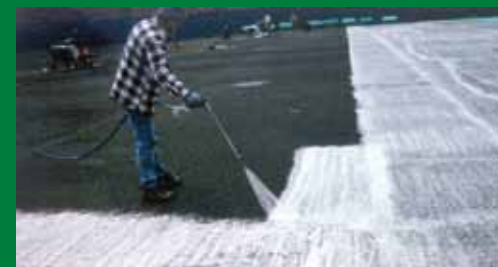
Spraying glue on asphalt for turf bonding
