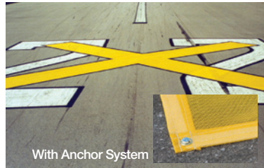
Runway Closure Marker With Anchor System
