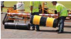
During winter storms, crews work 12-hour shifts around the clock.
