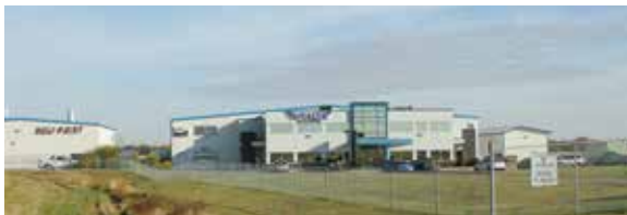
Recent airfield improvements include new hangars, aircraft services and runway extension.
