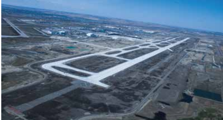
Calgary International Airport (YYC) Runway Development — Calgary, Alberta, Canada
