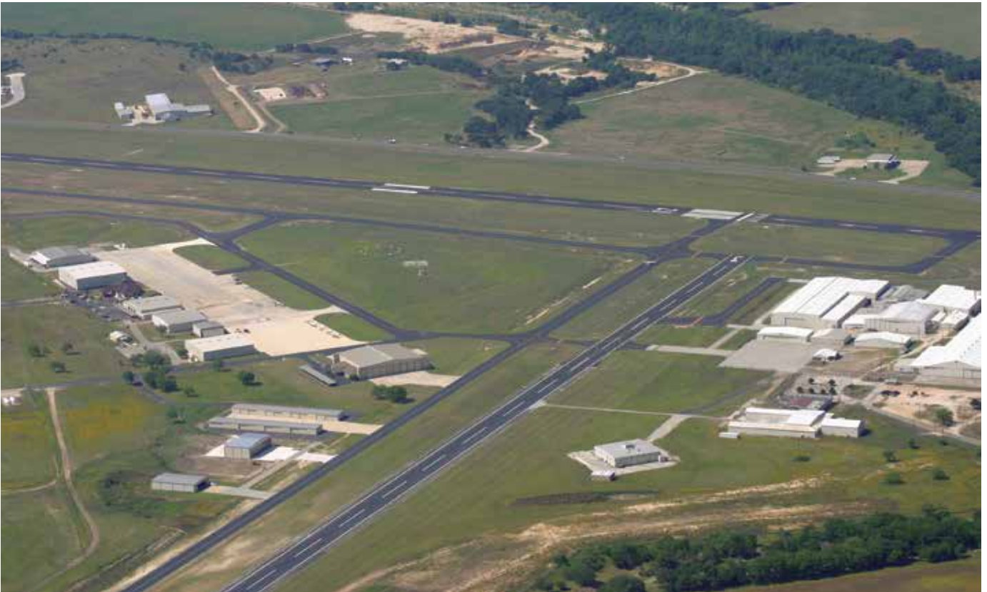
The airport's additional hangars are expected to generate about $46,800 of new revenue per year.
