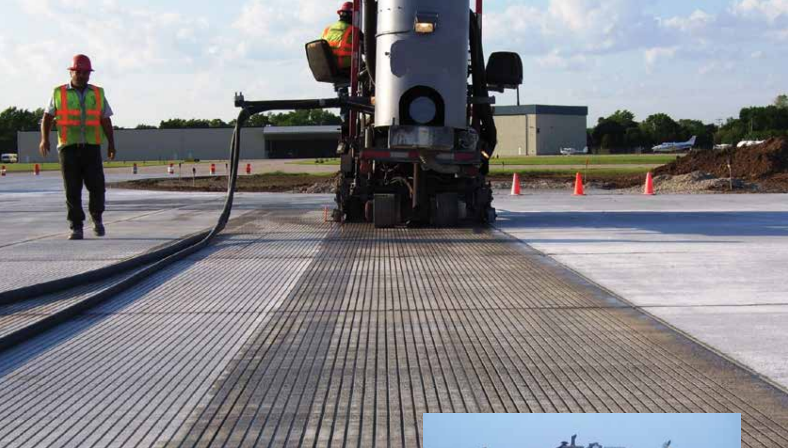
The airport allowed the asphalt on Runway 7-25 to cure for a full year after its last renovation before adding grooves.
