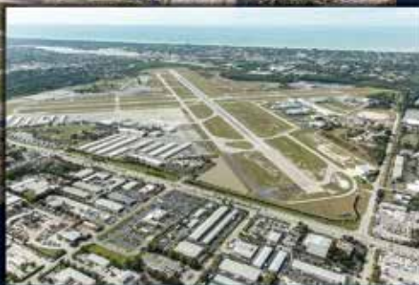
Taxiway A extension and water management system improvements, planning, design, permitting and construction Naples Municipal Airport Naples Airport Authority, Florida
