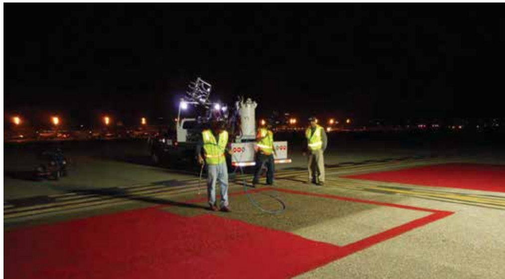
Despite the tight schedule, crews took time for surface preparation.
