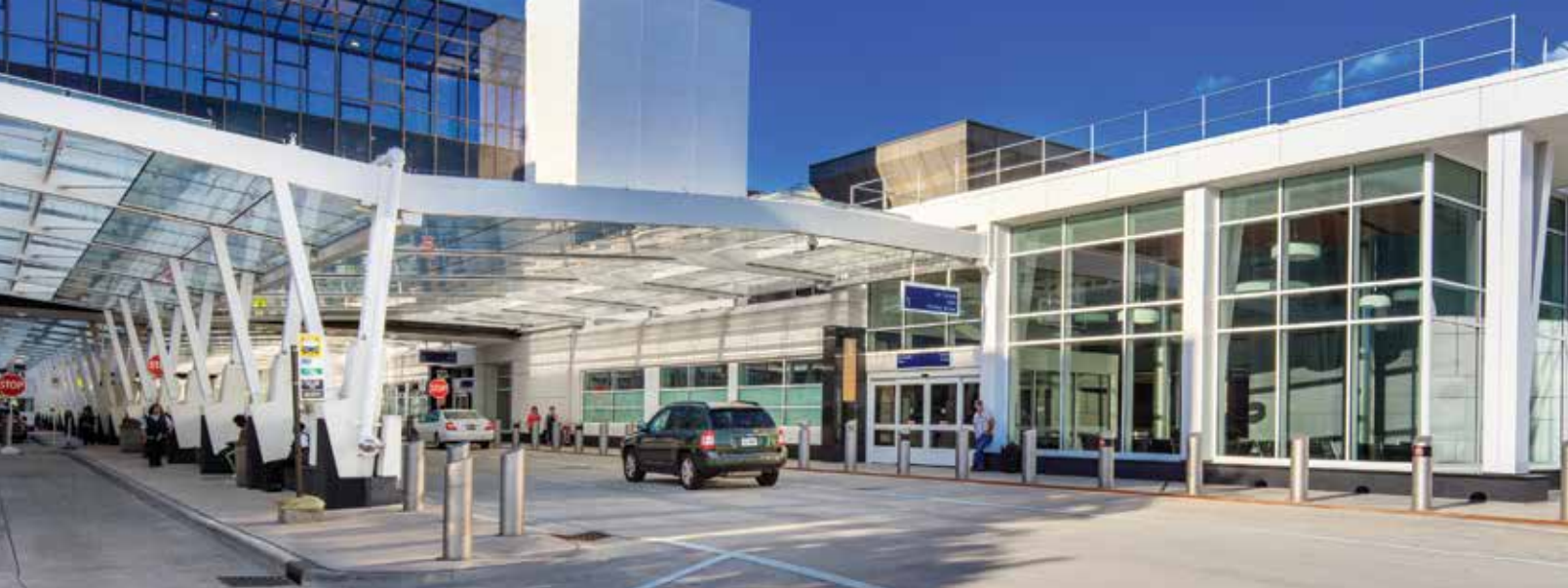
A glass canopy between the parking garage and new baggage claim building helps protect visitors from inclement weather.
