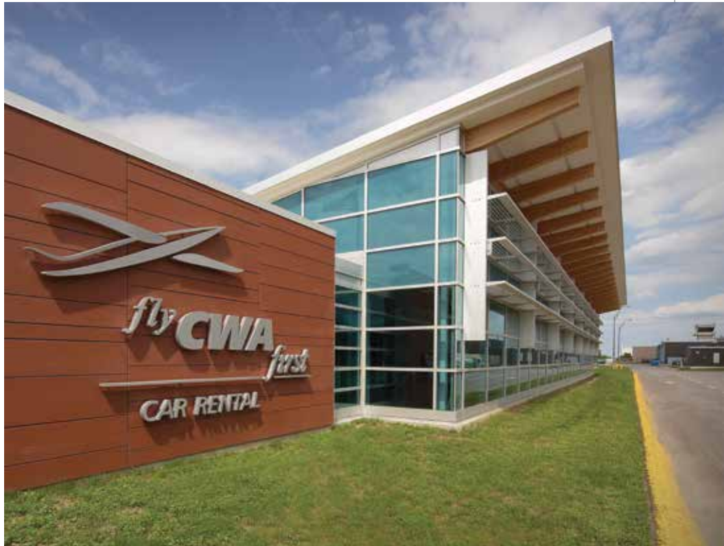
36 Five-Year Terminal Renovation Worth the Wait for Central Wisconsin Airport
