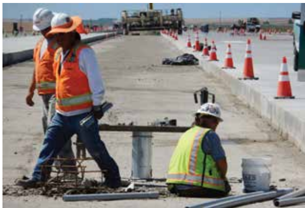
Active sensors, above, are a crucial component of the airport's new ice warning system from ASFT.
