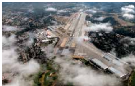
56 Monterey Regional Adds Runway Safety Areas Amid Perfect Storm
