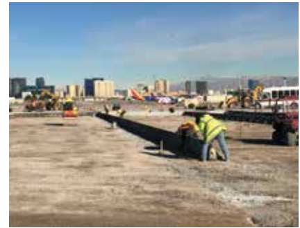
34 McCarran Int'l Completes Transition to All-Concrete Runways
