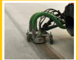
Curing Compound Removal
