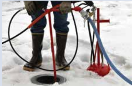
Left: An evacuation wand clears ice, melting water and other extra materials from the can. Right: Close-up of partially completed clearing process.
