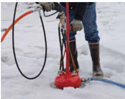
26 Alaska Tries New Method for Repairing Runway Lights
