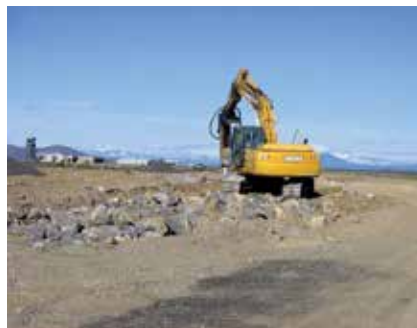
42 Redmond Municipal Mitigates Impact of 3-Week Closure
