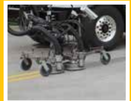
Car Park Marking Removal
