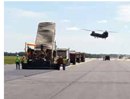
46 Reconstructed Runway Rises From Rubble at Coles County Memorial
