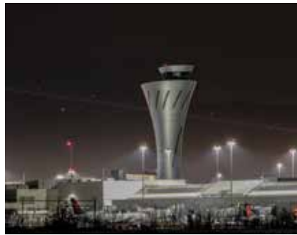
14 San Francisco Int'l Makes a Design Statement With New Control Tower
