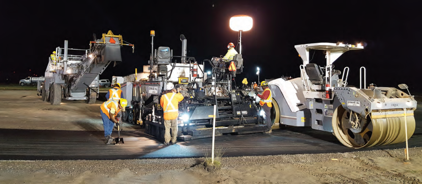
Crews resurfaced the entire runway during the airport's overnight curfew period.
