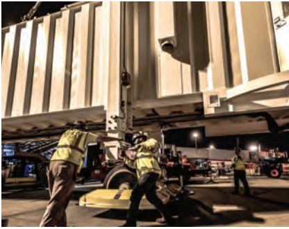
8 Atlanta Int'l Tackles Nation's Largest Ground Support Project
