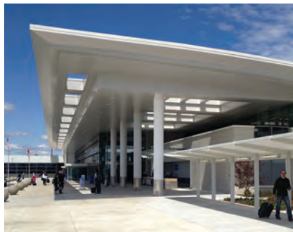
14 Clinton Nat'l Stresses Passenger Comfort in Terminal Improvements
