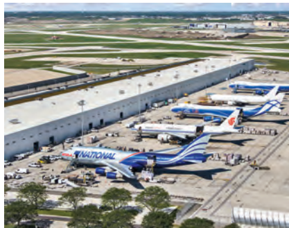
32 O'Hare Int'l Continues to Expand Cargo Capacity With New Landside Warehouse
