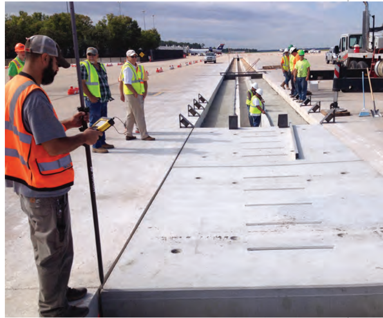
Manhole access points were installed every 300 feet to facilitate maintenance.
