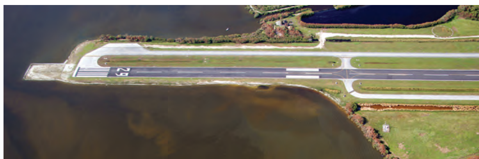
62 Merritt Island Airport Builds Seagrass Island, Restores Saltwater Marsh to Add New Runway Safety Area
