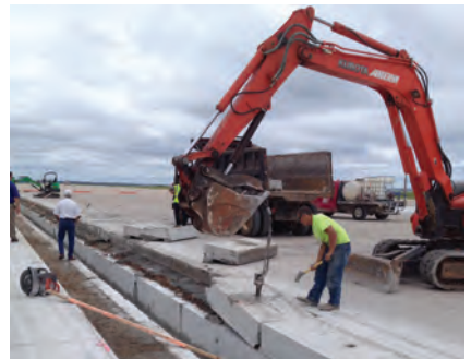
36 Greenville-Spartanburg Int'l Installs Concrete Trench Drain
