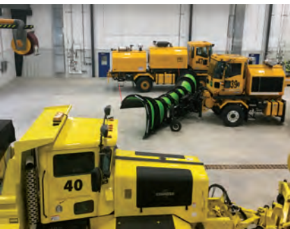
40 Casper Int'l Builds New Equipment Storage & Maintenance Facility
