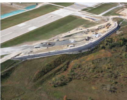
34 Wetlands & Wildlife Complicate Instrument Landing System Project at Worcester Regional
