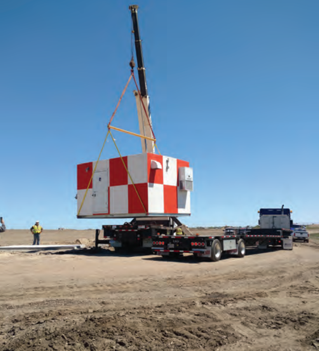
Beyond pavement, the project included new lighting and perimeter fencing.
