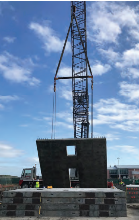
Despite setbacks from Hurricane Florence, construction was completed in September 2018.
