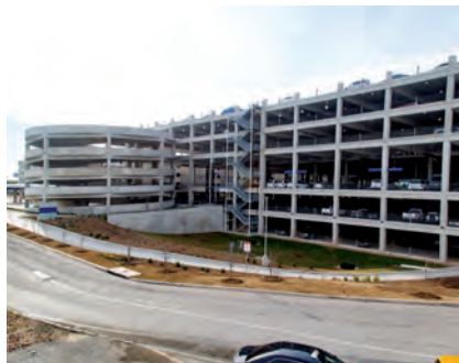
12 San Antonio Int'l Builds Consolidated Rental Car Facility & New Parking Garage
