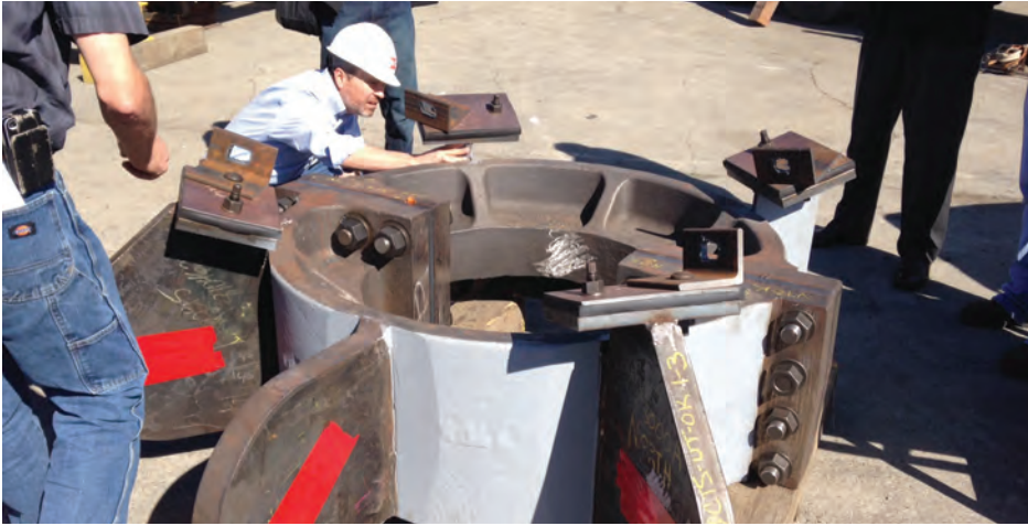
Using prefabricated cast steel column collars helped reduce disruptions inside the terminal during installation.
