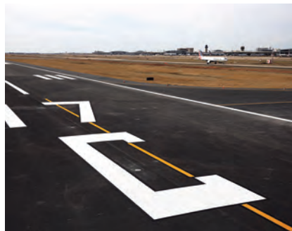
32 Dallas Fort Worth Int'l Rehabs Primary Arrivals Runway With Asphalt Overlay
