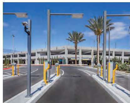
50 Innovation Lab at San Diego Int'l Tests Potential Parking Solutions
