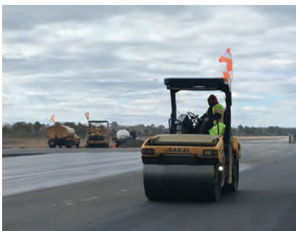
44 Island Location Complicates Runway Project at Martha's Vineyard Airport
