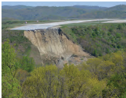
8 Yeager Airport Rebuilds Runway Safety Area After 2015 Landslide
