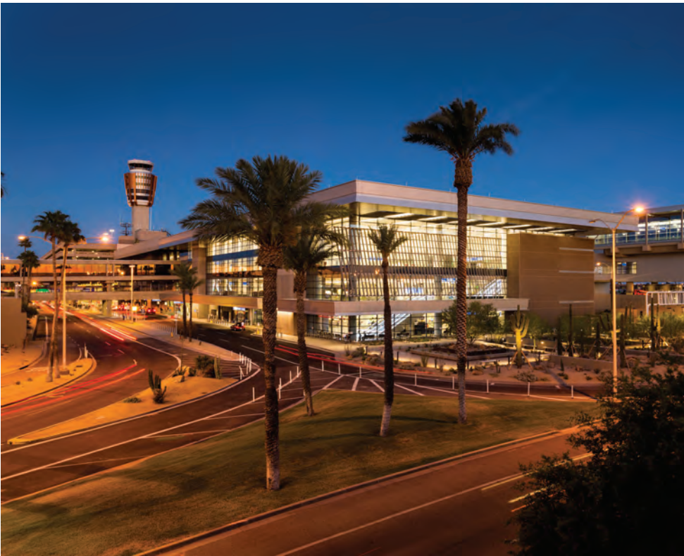
8 Transformation of Terminal 3 at Phoenix Sky Harbor Finishes with North & South Concourses
