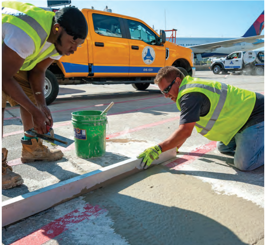
Crews repair pavement and apply new markings during warmer months.
