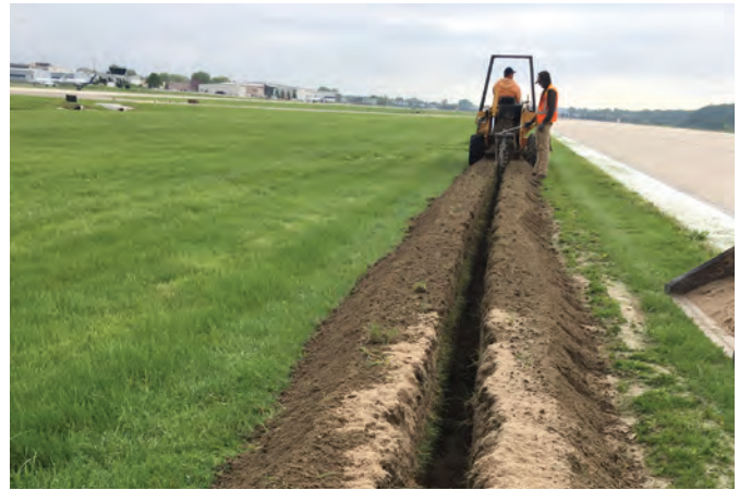
Workers trenching in new high-intensity edge lights for the main runway.
