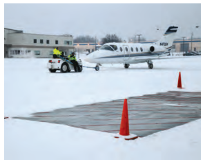
46 Test Slabs at Des Moines Int'l Bode Well for Electrically Heated Airside Pavement
