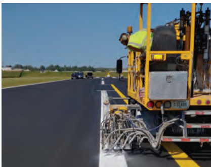
30 DeWitt Spain Airport Applies Sealcoat to Preserve New Runway Asphalt
