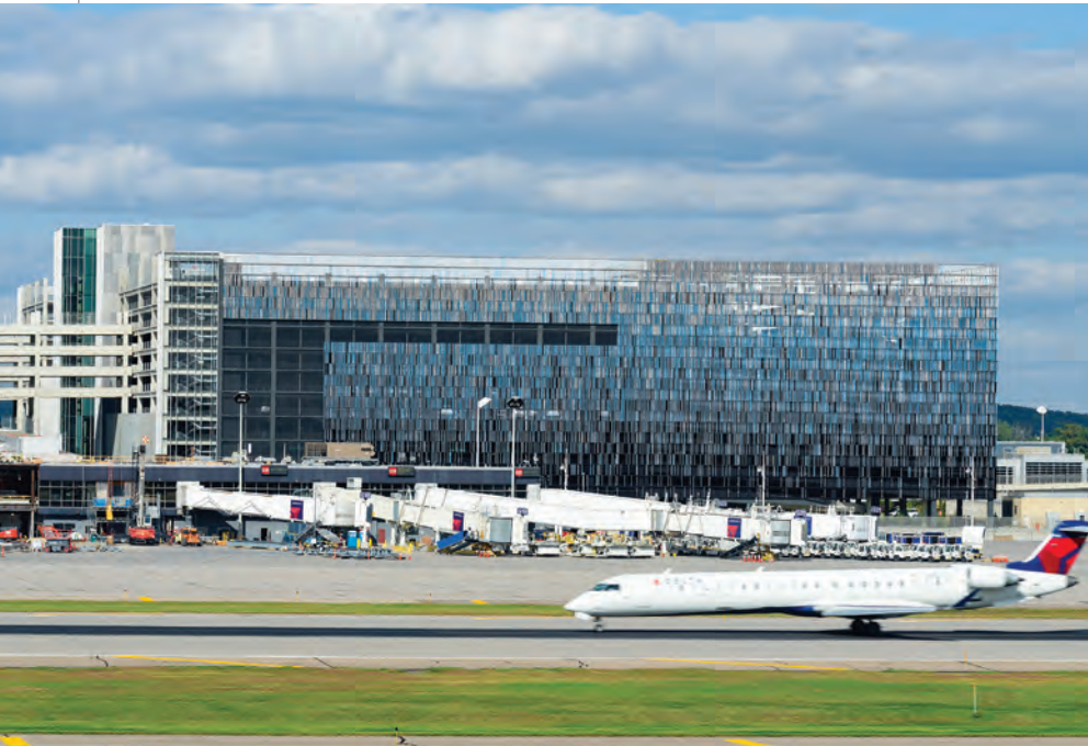
Designers specified terracotta baguettes on the airfield façade to prevent interference with navigation communications.
