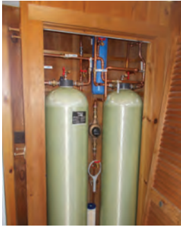
The airport has spent about $2 million on the PFAS issue, including point-of-entry water treatment systems (shown left) for some nearby homes and a remediation system (shown right).
