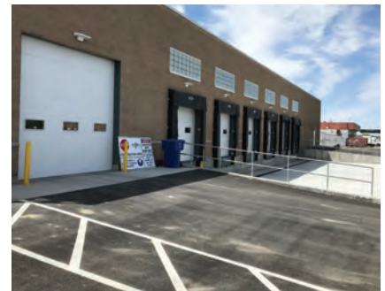
48 New Receiving & Distribution Center Improves the Way Goods Move Through Salt Lake City Int'l
