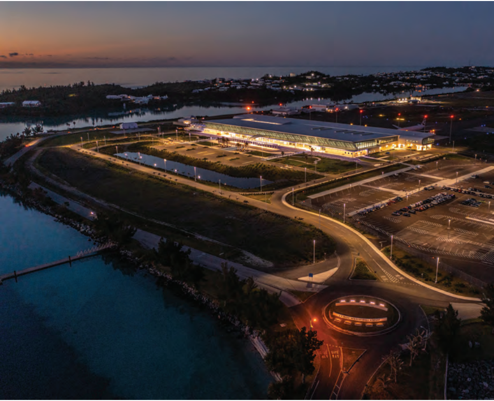
8 Public-Private Partnership Delivers New Terminal in Bermuda
