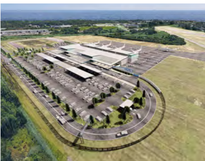
46 Tweed-New Haven Regional Prepares for New Traffic With Funding From Avelo Airlines & Avports
