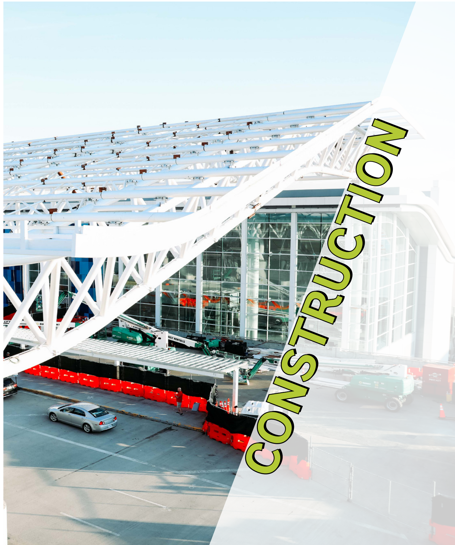
Terminal Lobby Expansion Canopy
