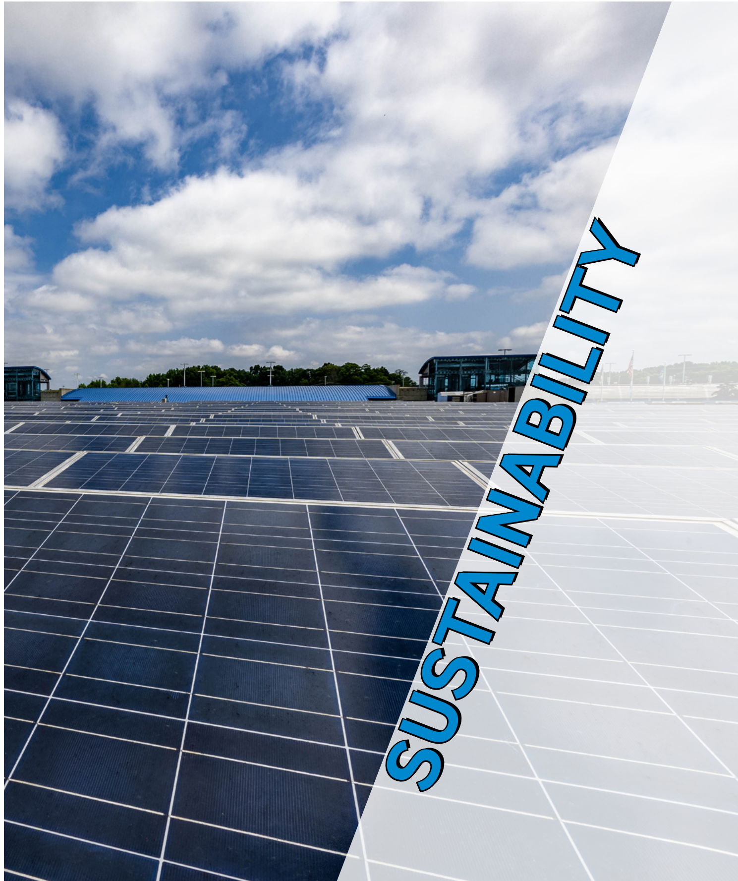
Solar Panels on CLT Center's Roof
