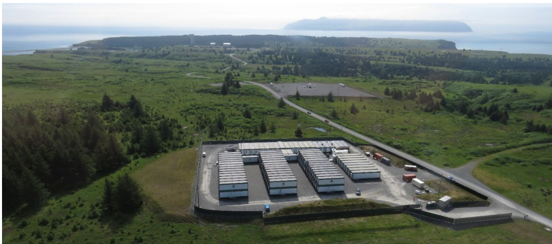
Figure 2-32: Area 4 Life Support Area (LSA) with Temporary Facilities
