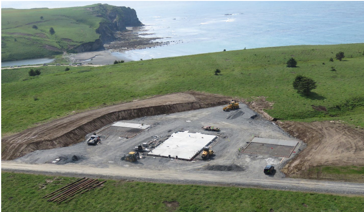
PSCA PAD 3B Construction Photo
