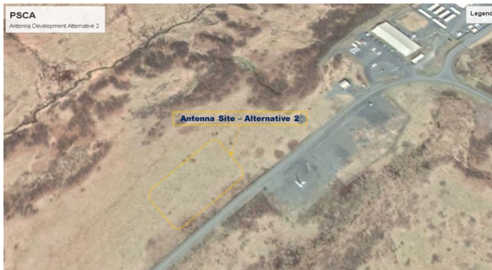
Figure 5-18: Telemetry Antenna Alternative 2 Site
