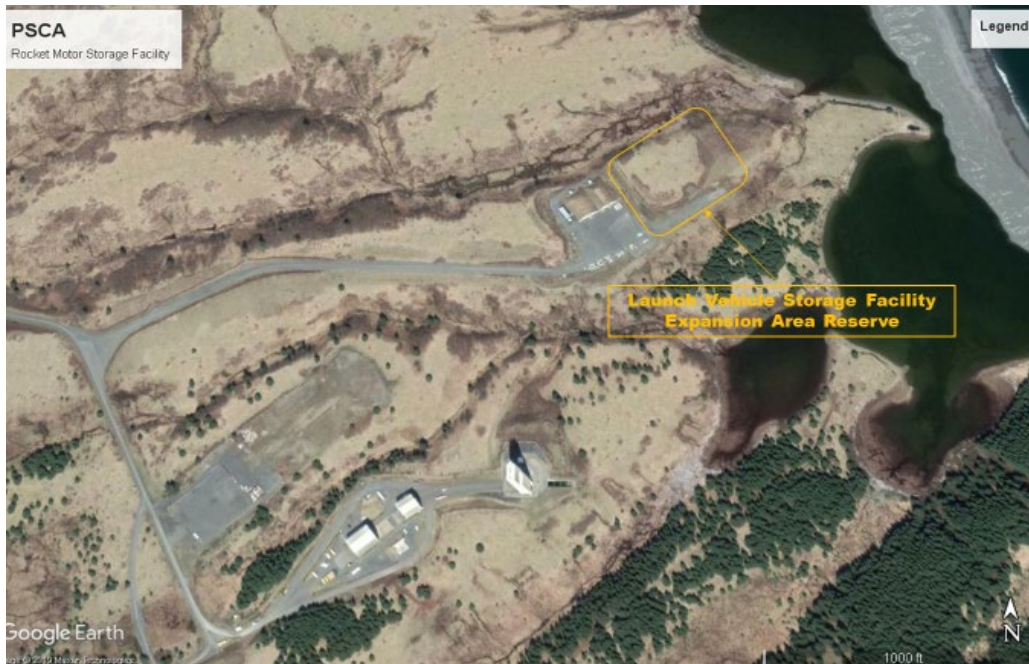
Figure 5-13: Launch Vehicle Storage Facility Expansion Area
