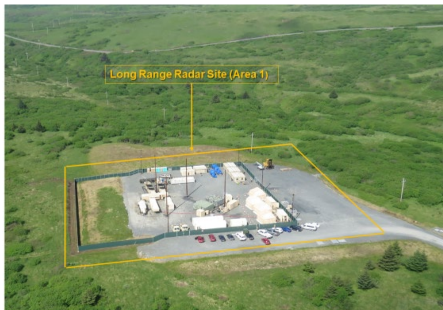
Figure 5-31: Long Range Radar Site (Area 1)
