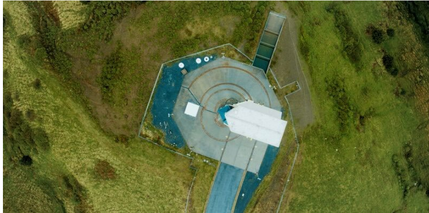
Figure 5-2: Overhead View of Launch Pad 1
