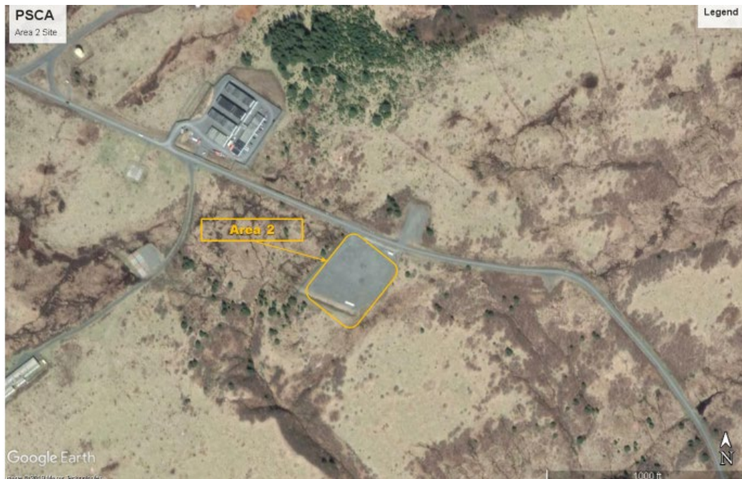
Figure 5-32: Radar Gravel Pad (Area 2)
