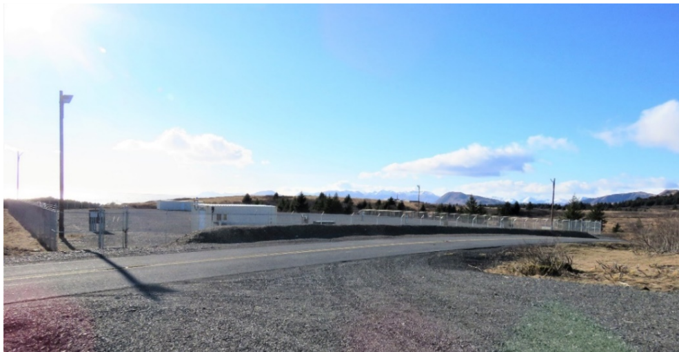
Figure 2-27. Area 2 Radar Site
