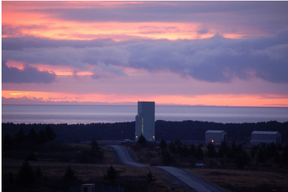
Figure 5-12: Launch Support Structure at Sunrise
