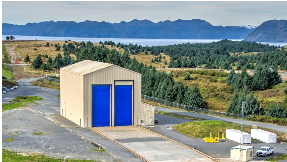
Figure 2-14: Integration and Processing Facility
