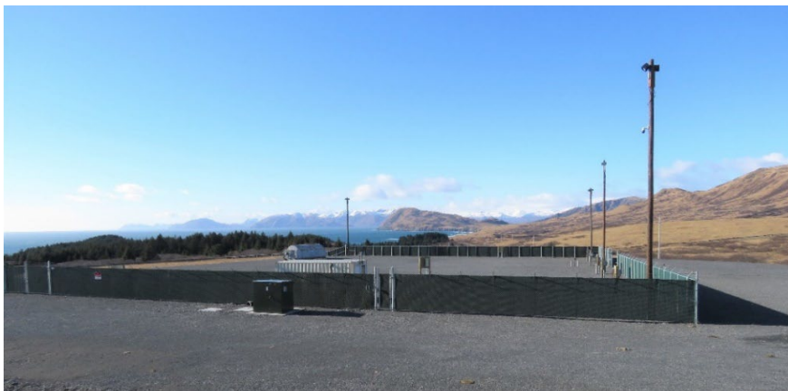
Figure 2-26: Area 1 Long Range Radar Site
