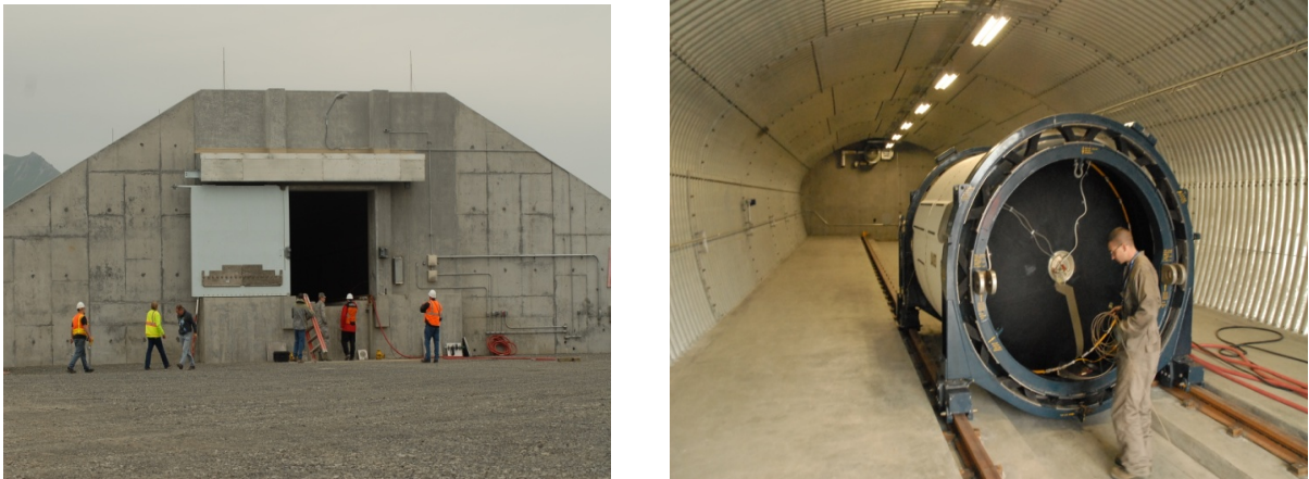
Figure 2-23: RMSF Storage Bunkers
