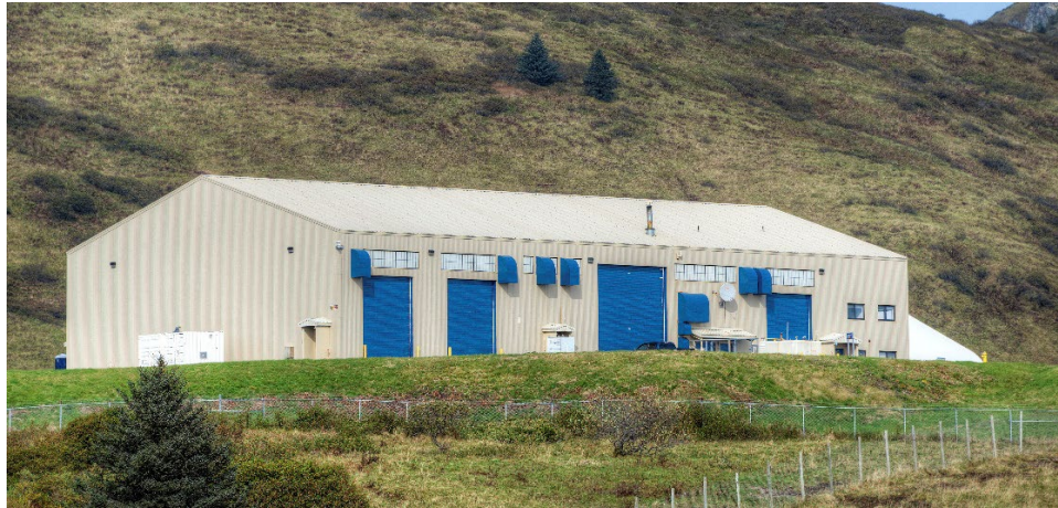
Figure 2-24: Maintenance and Support Facility (MSF)
