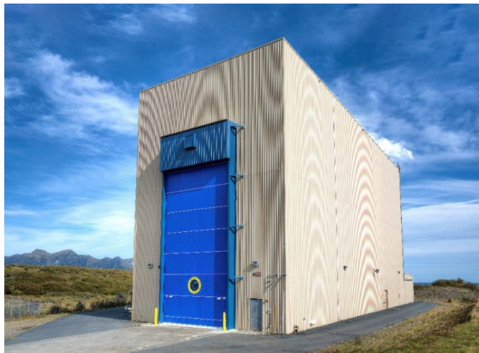
Figure 2-10: Payload Processing Facility
