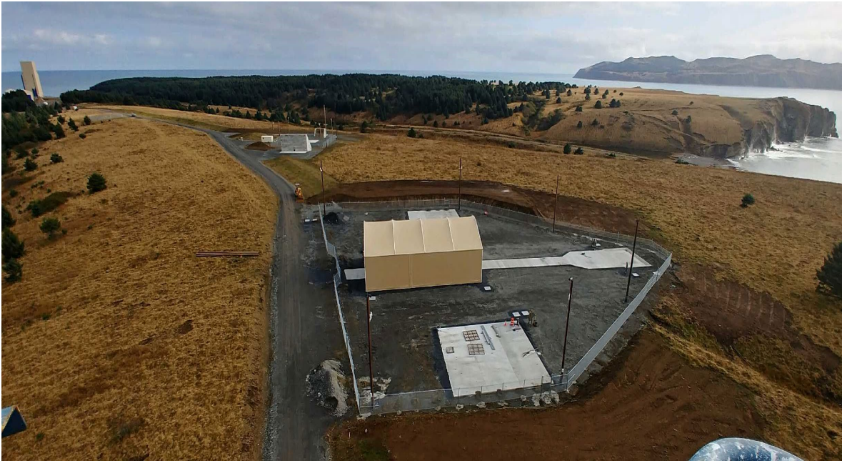
Figure 6-3: Pad 3B Aerial Photo with Pad 3C and LP1 tower in the background
