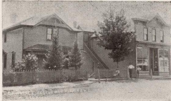
RESIDENCE AND STORE OF P. J. HEINTZ, LEOPOLIS, WISCONSIN.
