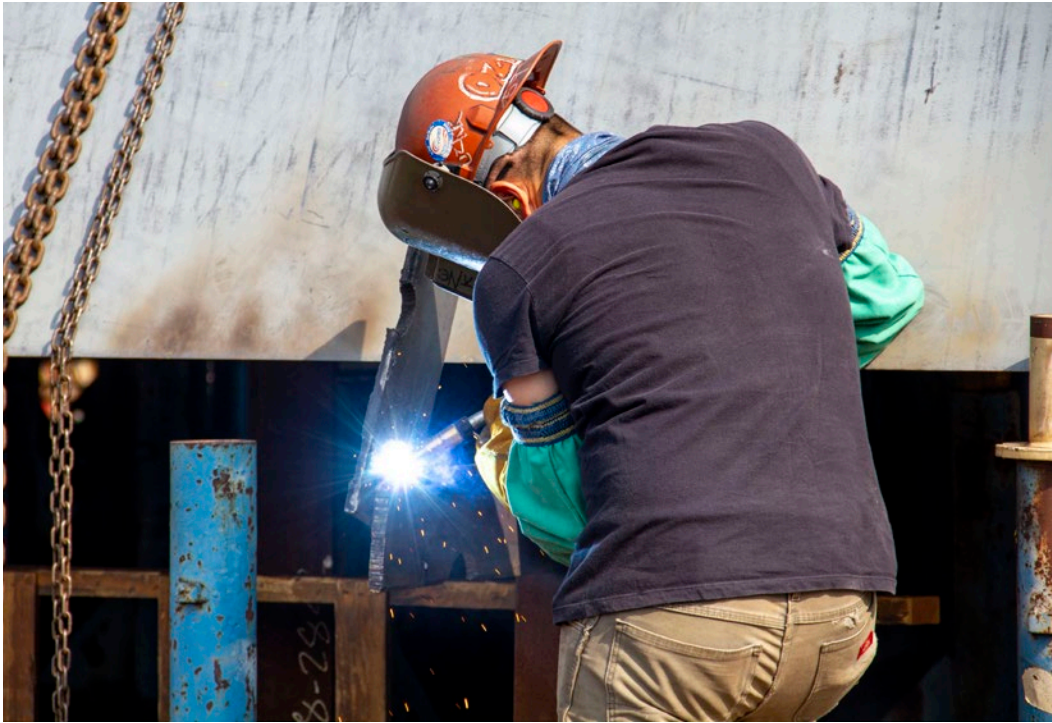
Employee welding at NASSCO
