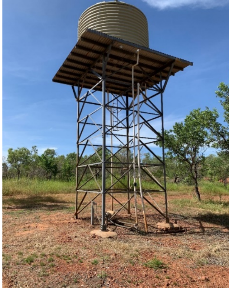
Figure 10: This water tower at Garlburang has no safety rail around its platform or the means to safely access it. We visited Garlburang, a very small East Kimberley community where the Department has no plans to improve or upgrade essential services, early in 2020
