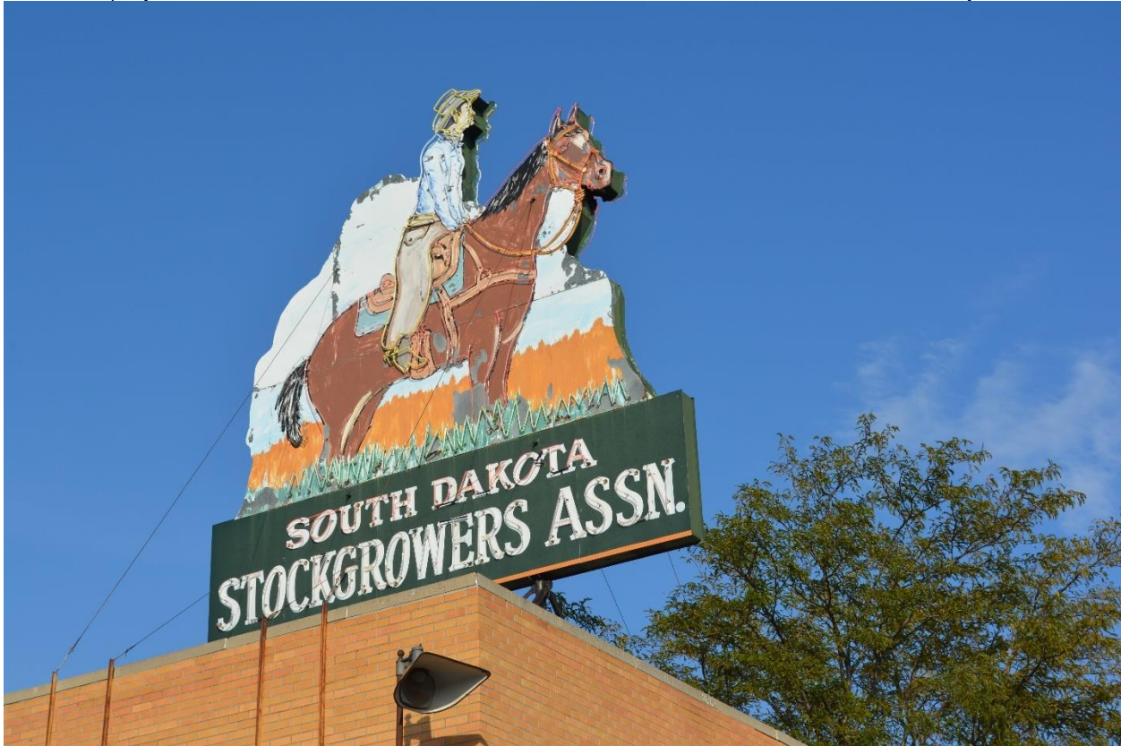
SD_PenningtonCounty_SouthDakotaStockgrowersAssociationBuilding_0007. Looking NE at roof.
