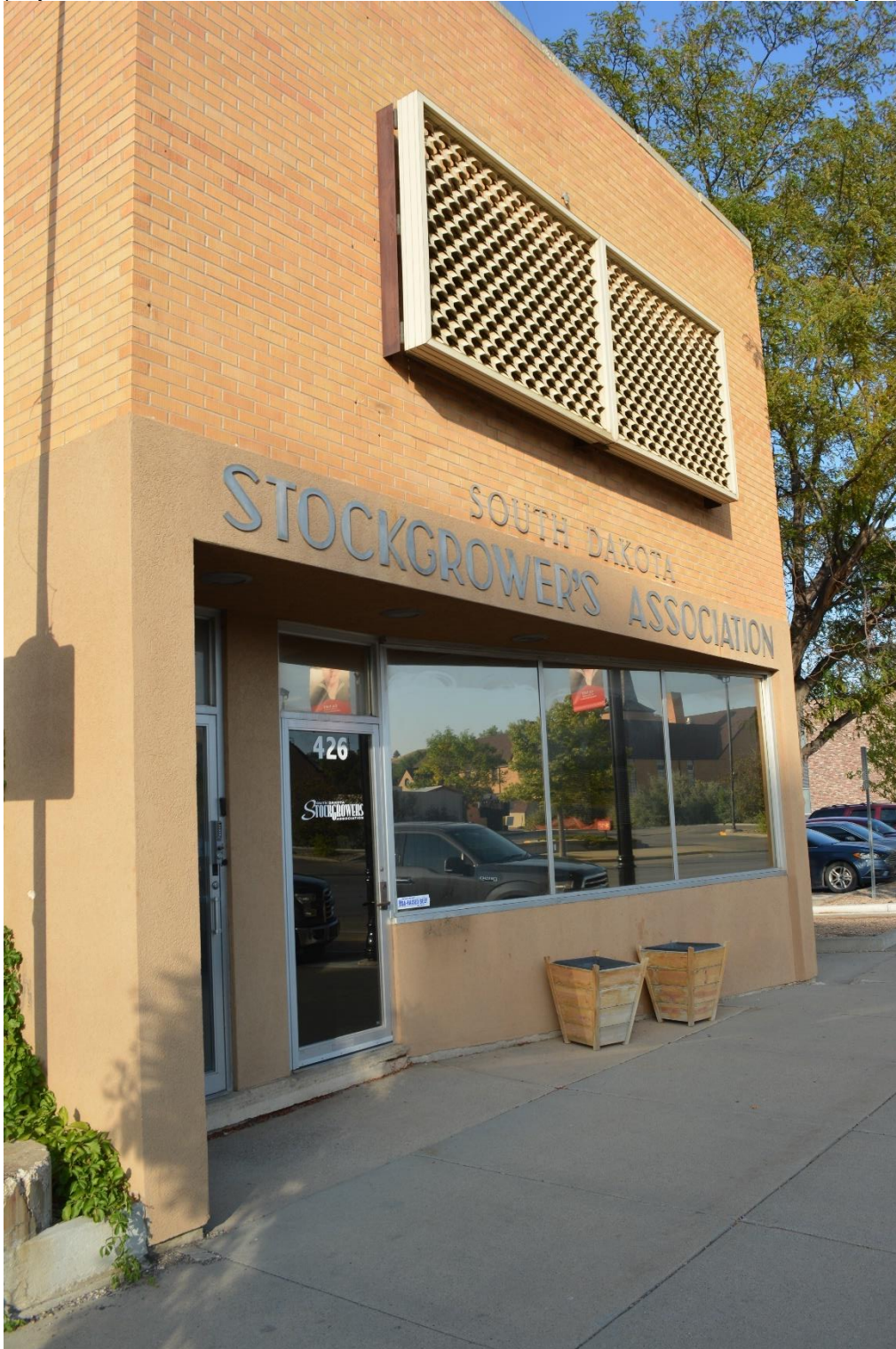
SD_PenningtonCounty_SouthDakotaStockgrowersAssociationBuilding_0006. Looking NE at the south (front) elevation.
