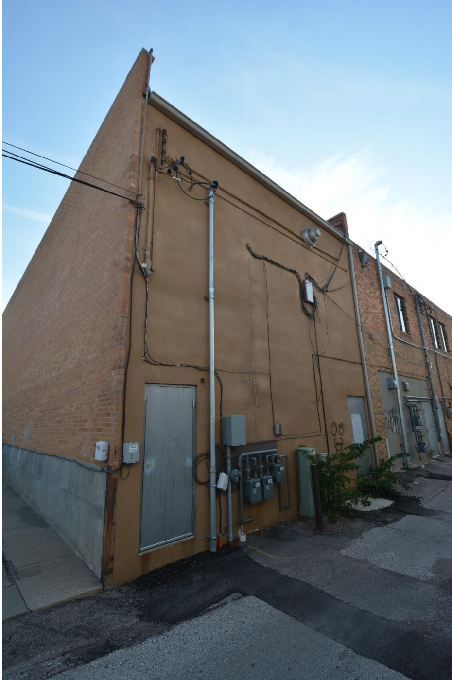
SD_PenningtonCounty_SouthDakotaStockgrowersAssociationBuilding_0004. Looking SW at the north elevation (rear).
