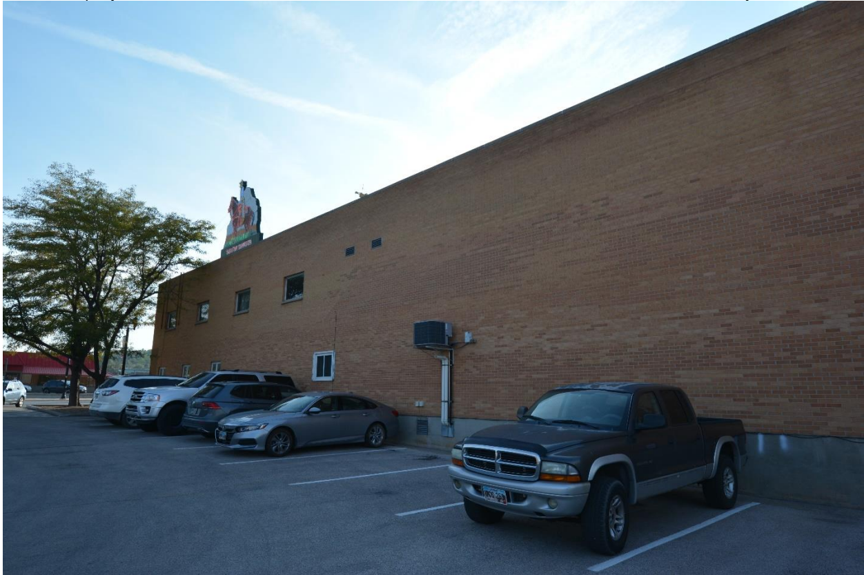
SD_PenningtonCounty_SouthDakotaStockgrowersAssociationBuilding_0003. Looking SW at the east elevation.
