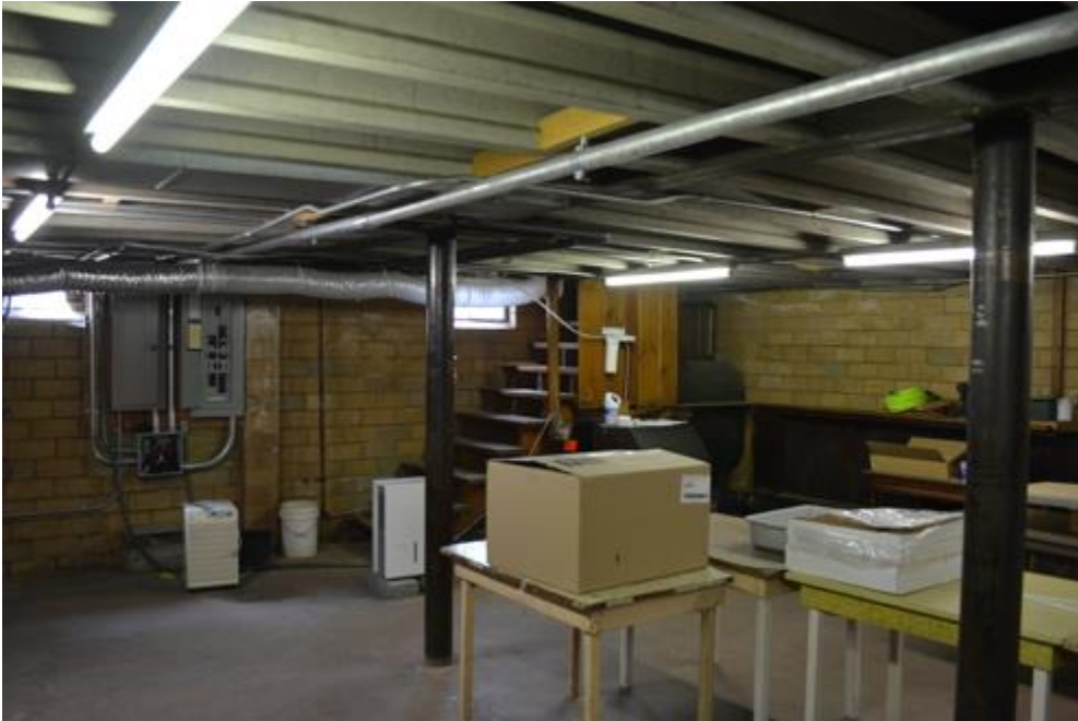
SD_BonHommeCounty_BesedaHallSokolPark_0018 View of lobby basement, camera facing northeast.
