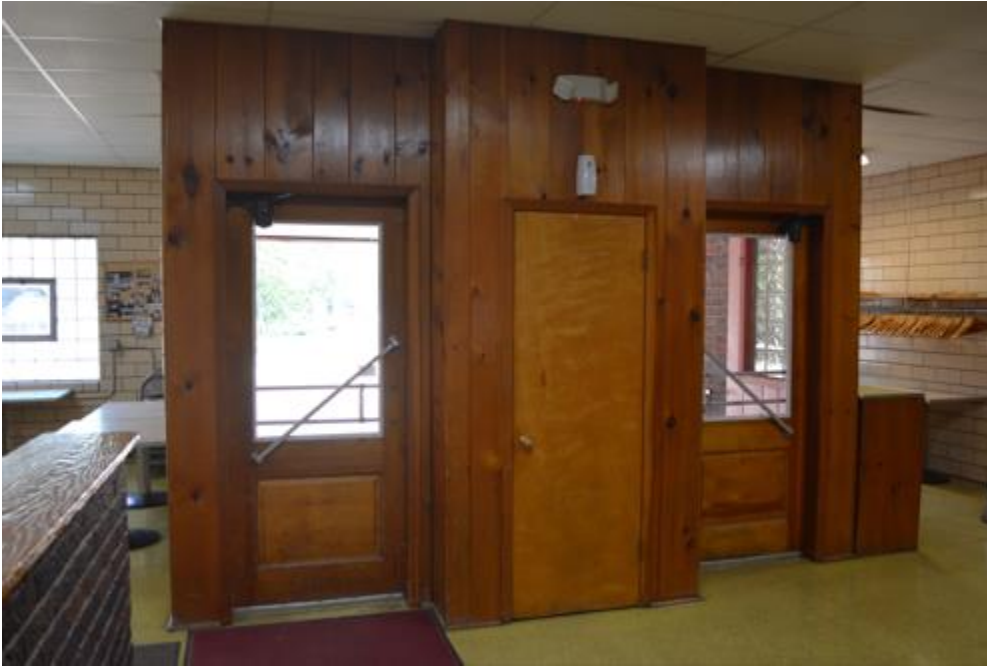
SD_BonHommeCounty_BesedaHallSokolPark_0012 View of lobby entrance, camera facing west.
