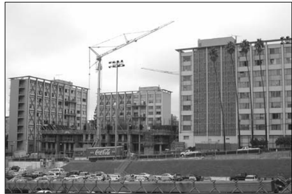
Residence halls with new construction underway fall 2003
