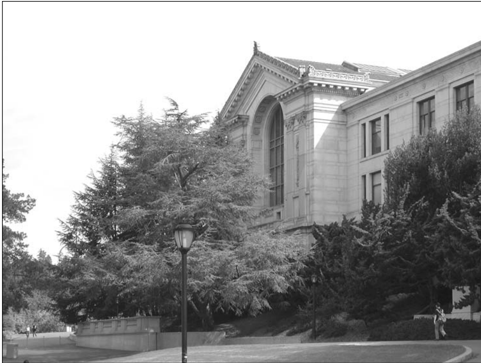
DOE LIBRARY FROM CAMPANILE WAY
