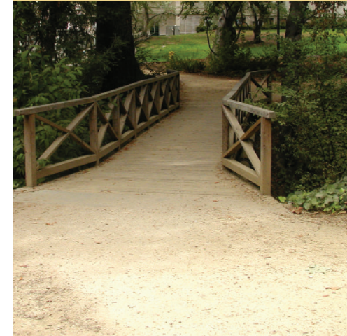
Example of a decomposed granite trail leading to a wooden bridge in the natural area along Strawberry Creek (2003).
