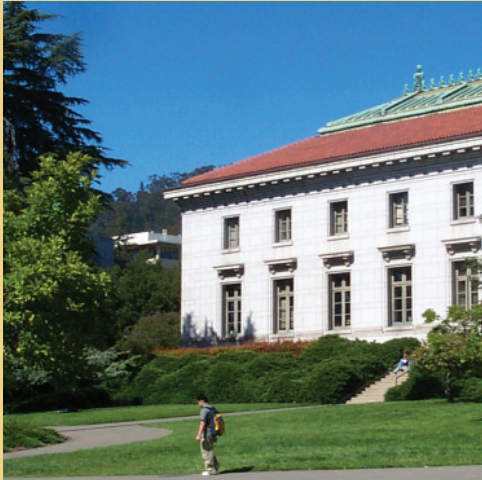
Example of typical landform creating a building terrace (2003).
