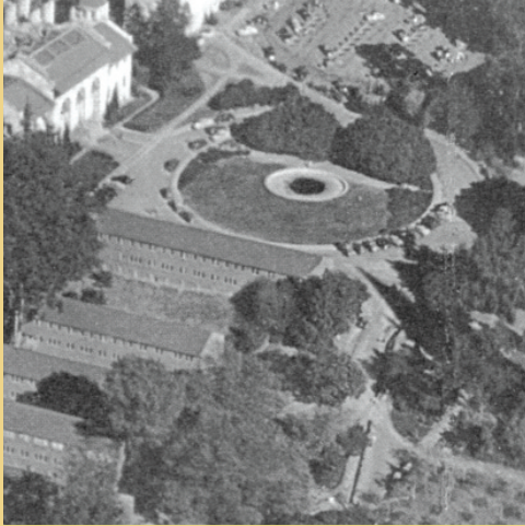
Temporary wooden buildings located west of Mining Circle (ca. 1949).
