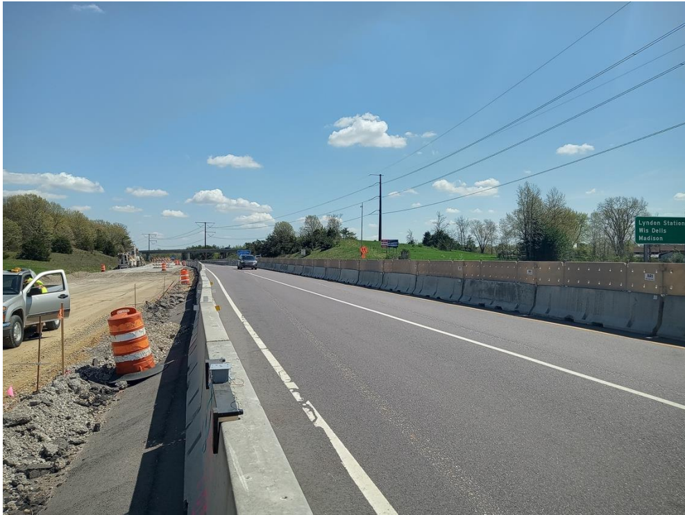
(a) Viewing upstream
