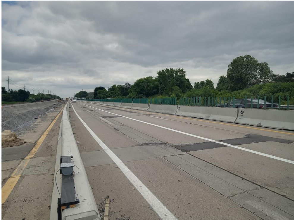
(a) Viewing upstream
