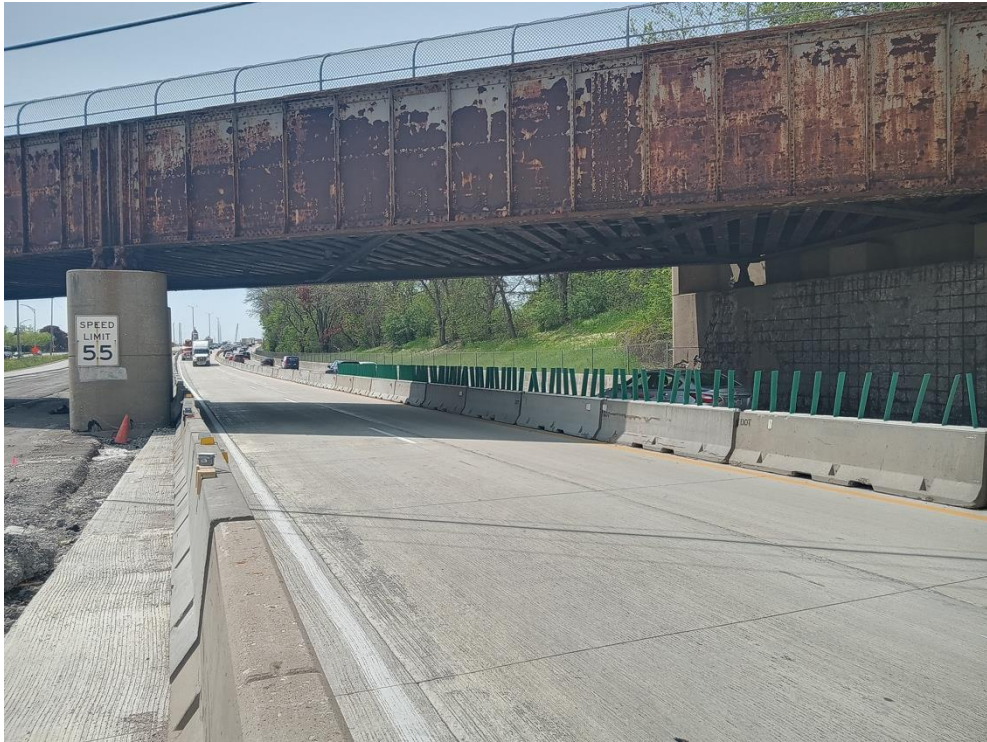
(a) Viewing upstream
