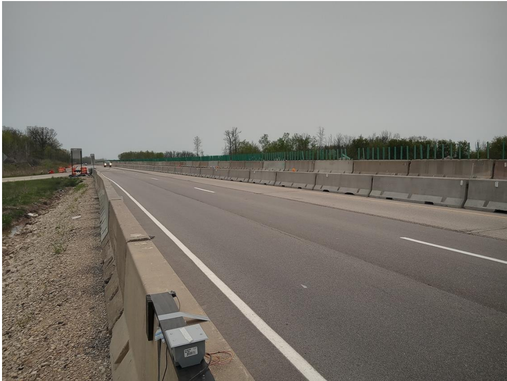
(a) Viewing upstream
