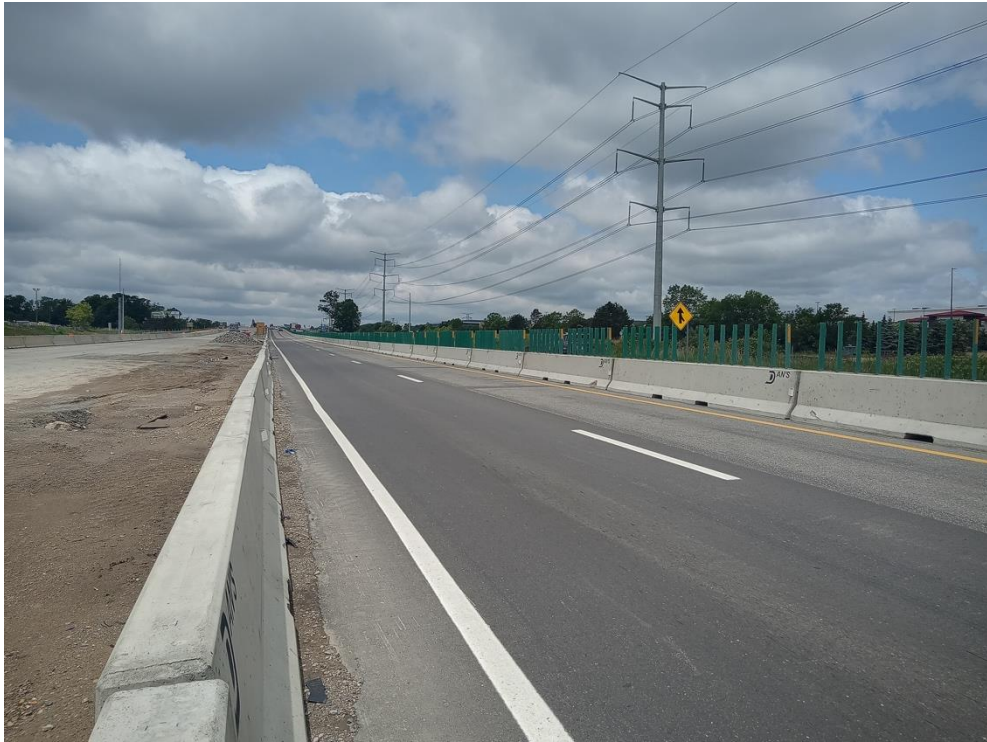
(a) Viewing upstream
