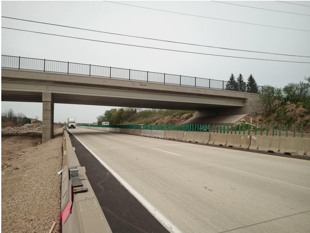
(a) Viewing upstream
