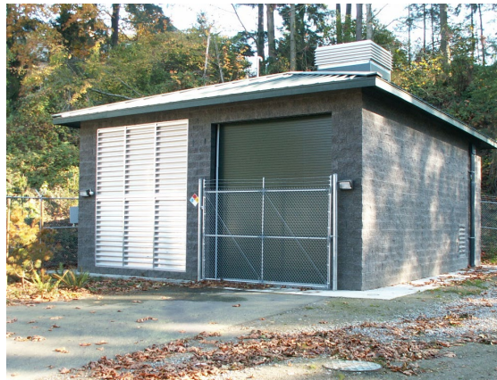
Mt. Olivet Booster Pump Station
