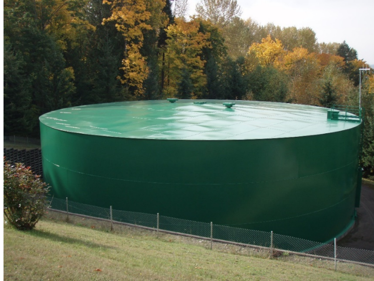
South Talbot Reservoir – 1.5 MG
