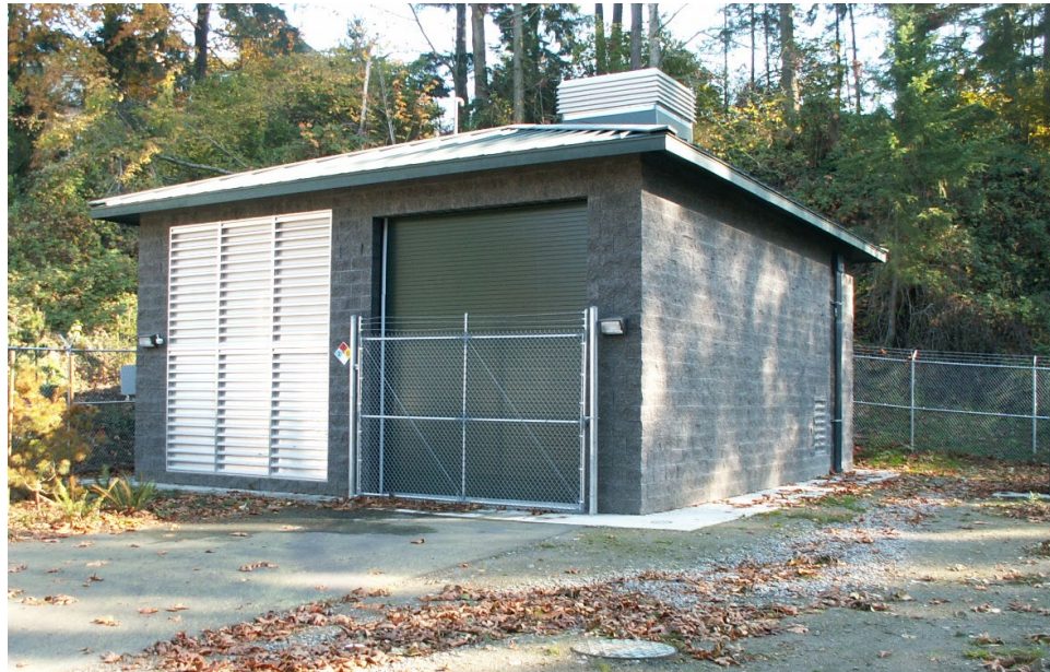
Mt. Olivet Booster Pump Station
