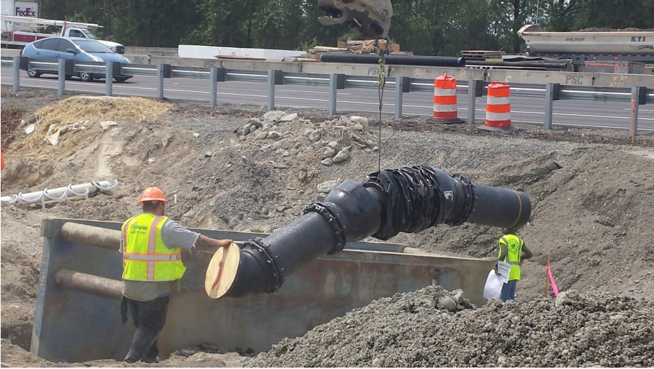
Pipeline -Flex Joint Installation
