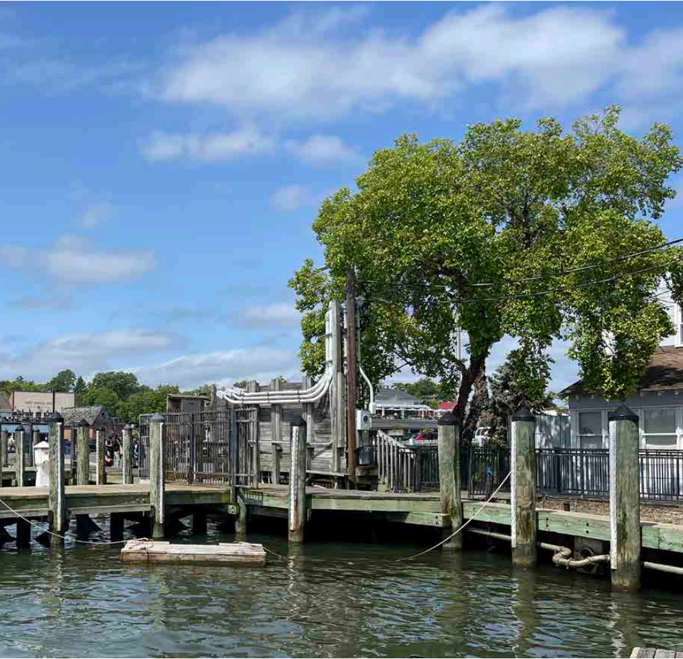
Existing View One
