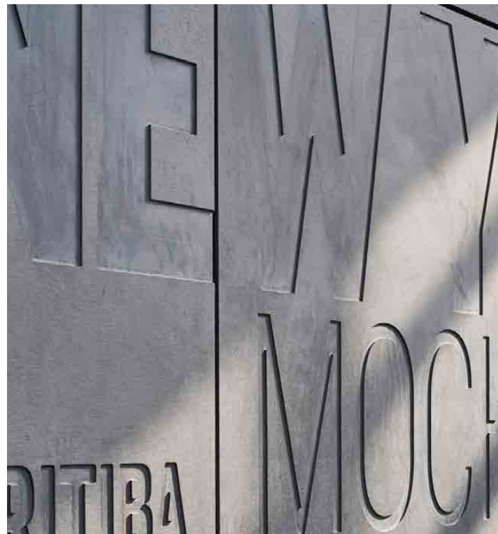
Fiber Cement Panel, Engraved Equitone Tectiva 12mm Panels, TE15
