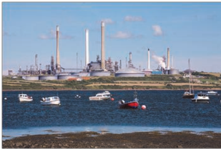
Milford Haven Refinery
