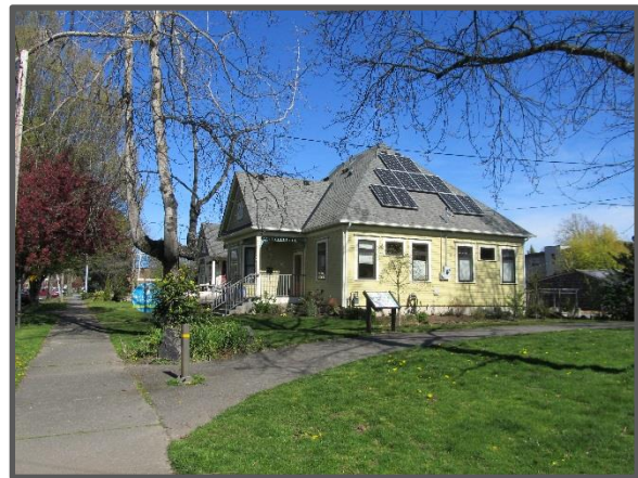
Solar panel retrofit on building near Old Village Trail.
