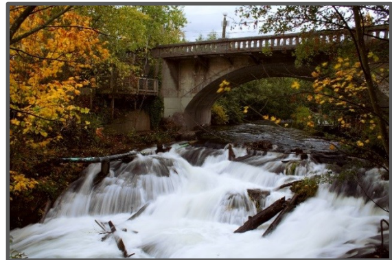
The Picket Bridge over Whatcom Creek opened in 1920 and was rehabilitated in 2002. Photo by Carey Thure.
