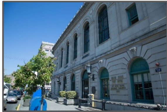
The Federal Building on Magnolia Street hosts a branch of the Post Office and City offices.
