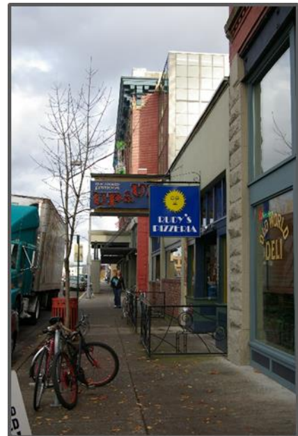
Mixed-use development on State Street, a WTA high-frequency transit route.
