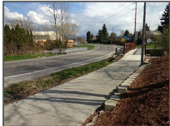
The Meador-Kansas-Ellis Trails project received a silver Greenroads certification. The project's sidewalks are composed of recycled toilets ("poticrete").
