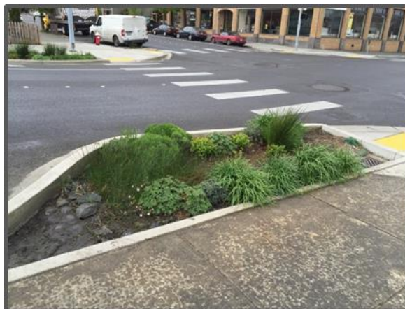
Installation of rain gardens downtown was coordinated with pedestrian improvements.
