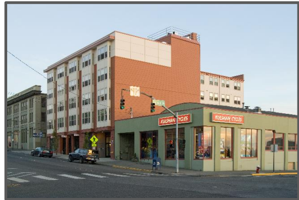
Kateri Court is a LEED-certified building consisting of commercial spaces and affordable studio and one-bedroom apartments.
