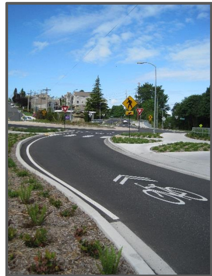
Wharf Street multi-modal roundabout serves as a gateway to several key locations.
