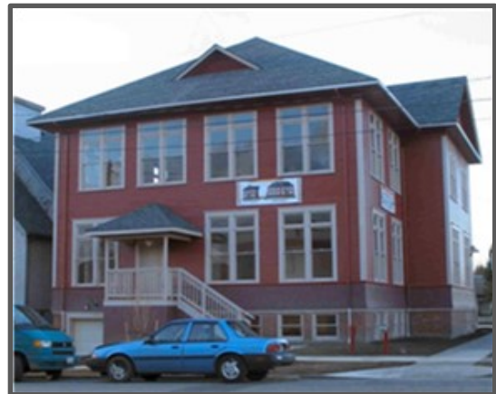
1303 Astor Street is listed on the National, State and Local Historic Registers.
