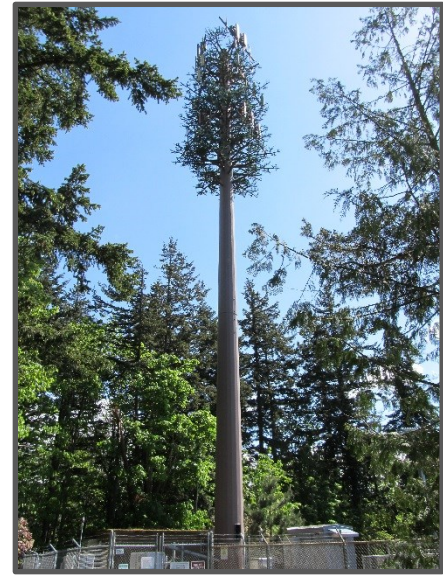
Concealed telecommunications monopole in the Happy Valley Neighborhood.
