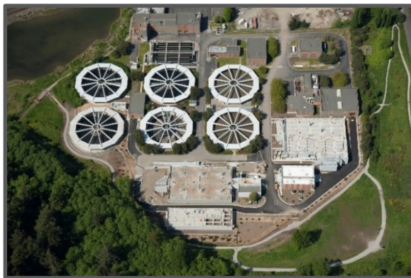
Post Point Wastewater Treatment Plant.
