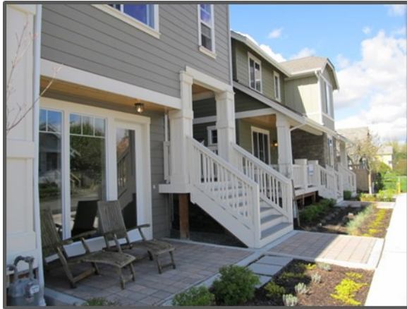
New townhomes on Peabody Street. Some units include an attached accessory dwelling unit.
