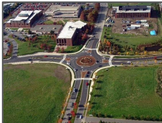
The multi-modal roundabout at Cordata Parkway and Kellogg Road was the first roundabout in the City (2002).
