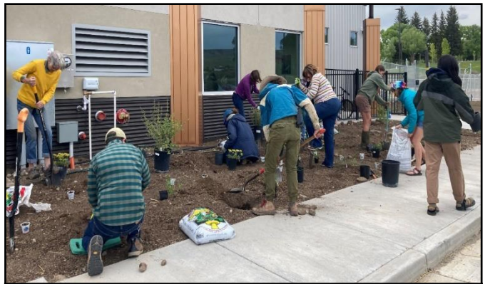
Workshop participants plant native plant species in the newly constructed BLM building's garden. © Marcella Tarantino, Bird Conservancy of the Rockies
