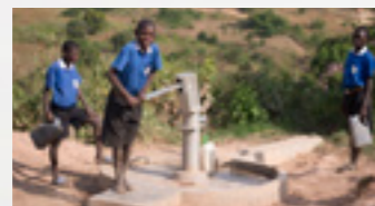
Boreholes, Rakai and Lwengo Districts, Uganda
