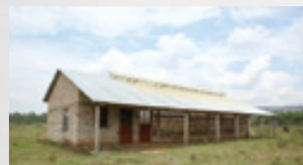
Coffee Drying Structures, Rakai District, Uganda
