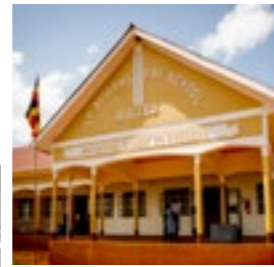
Busibo Secondary School, Lwengo District, Uganda 1,000 educational places
