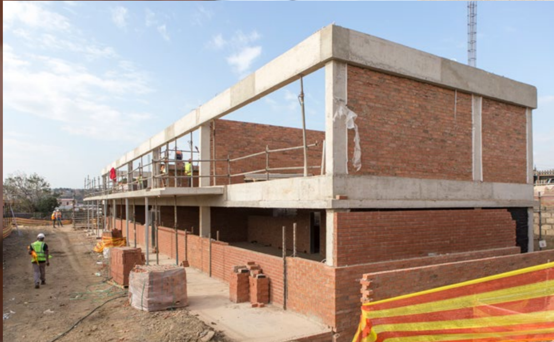
Dr JL Dube High School - under construction (opening in 2023)
