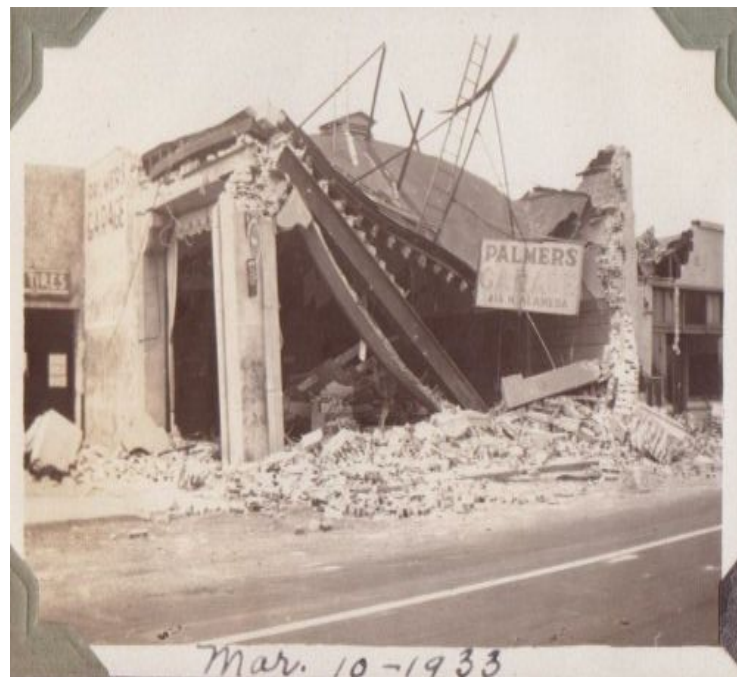
Figure 2-3. Damage to an unreinforced masonry building in the 1933 Long Beach earthquake. Source: USGS
