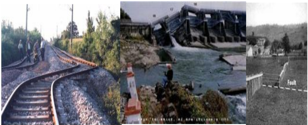
Figure 3-4. Three examples of fault crossing damage. The railway was bent when the fault in the 1999 Izmet, Turkey earthquake moved sideways (lower part of the picture to the left) about 7 ft. The dam was damaged when the 1999 Chi Taiwan earthquake moved (right side up) about 25 ft. The fence was broken when the 1906 San Francisco earthquake moved 5 ft.
