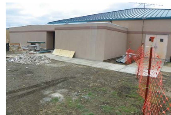
Excuse the mess while we finish renovation of the kitchen!
