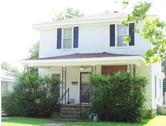
Repairs done on Sally Farley's house. Photo courtesy Dana Murrell.
