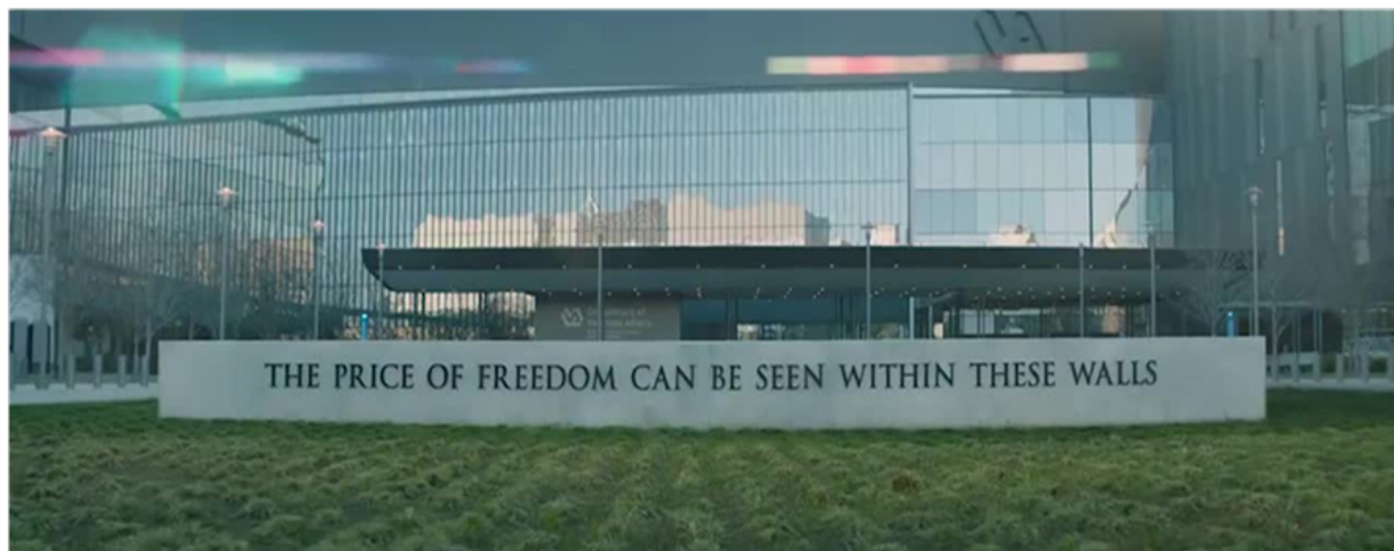
Figure 3. The New Orleans, Louisiana VA Medical Center.
